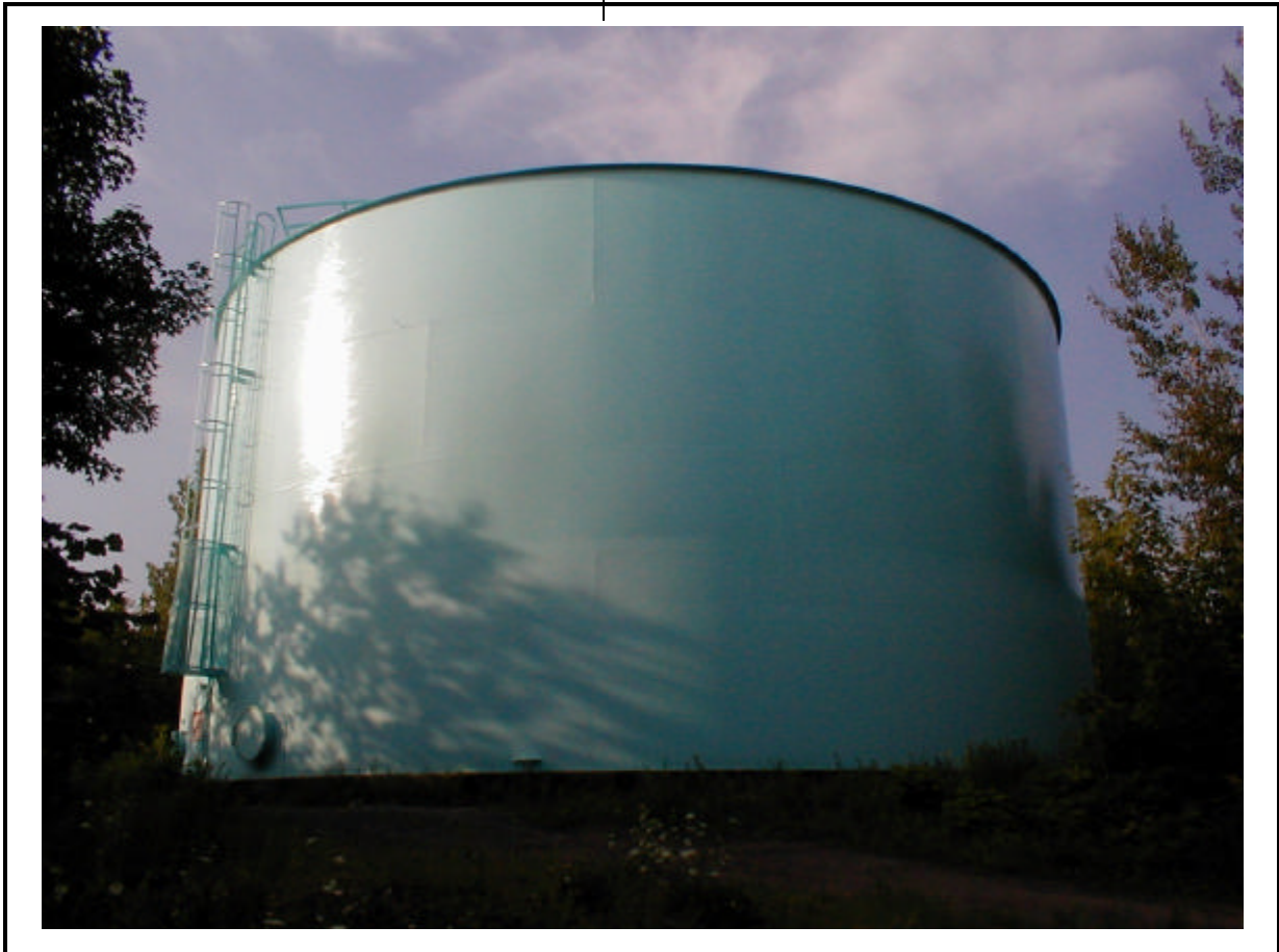
Marquette Township water tank located on Cox Avenue.
