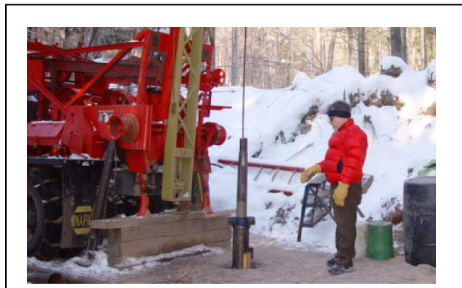
Kirk Page observing the drilling of the test well.
