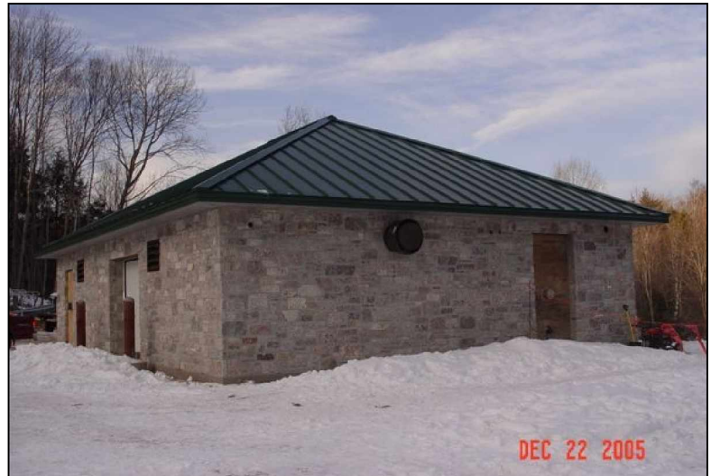
Well/Pump House nearing completion (December 22, 2005) looking northwest.
