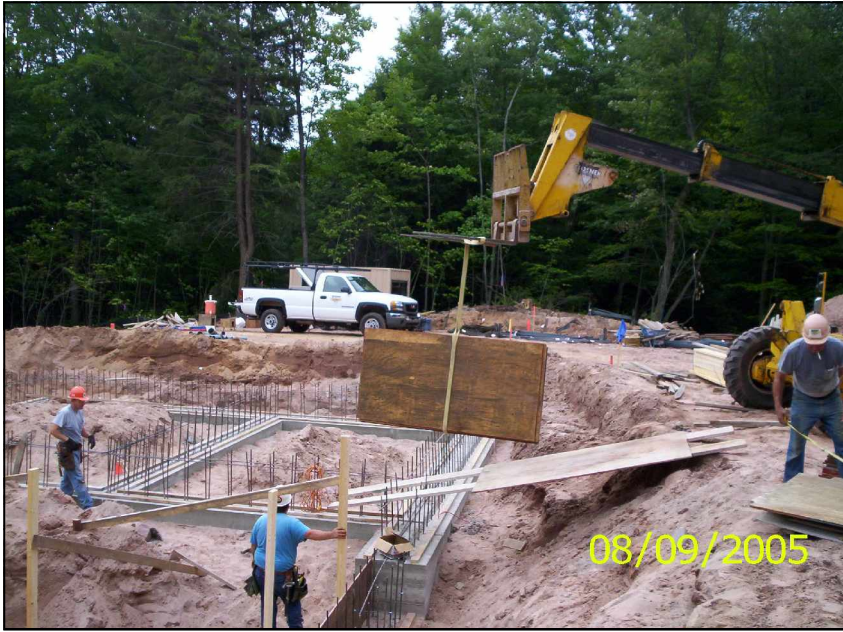
Construction of foundation for Well/Pump House (August 9, 2005).
